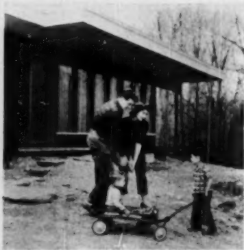
Mrs. Porter, once a student of design, planned the house. She and her husband, "helped" by their sons, did much of the work themselves
